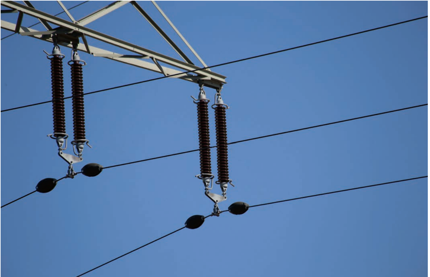
The wireless sensors below the insulators enable the monitoring of high and extra-high voltage lines. © Fraunhofer IZM
